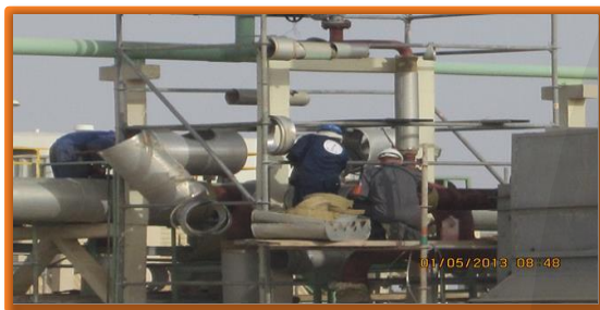
ZOC-103A REMOVING INSULATION FROM HOT LINES
