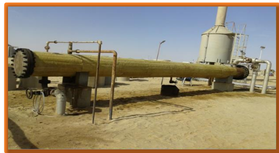
ZOC-103A INSTALLATION SLIP BLIND AT FLARE
