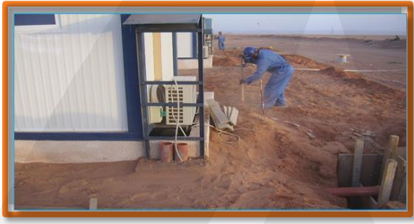
Hand digging and excavation works for UT survey
