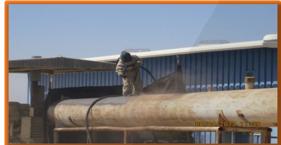
ZOC-103A – PRE-SHUTDOWN blasting /FUEL TANK
