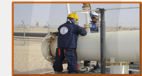
ZOC-103A/ INSTALLATION GATE VALVES WITH
