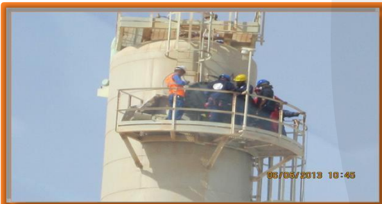
ZOC-103A/ INSULATION CLADDING AT F-12 HEATER
