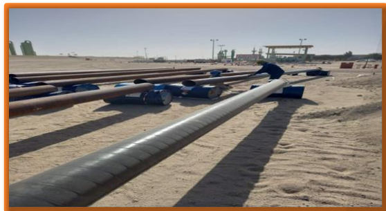
ZOC-103A INSULATION AND CLADDING AT F-12
