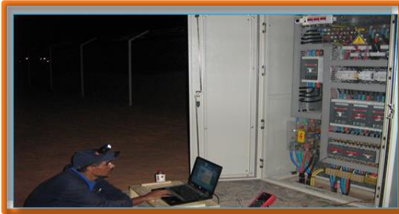
Electrical works mostly consisting of configuration
