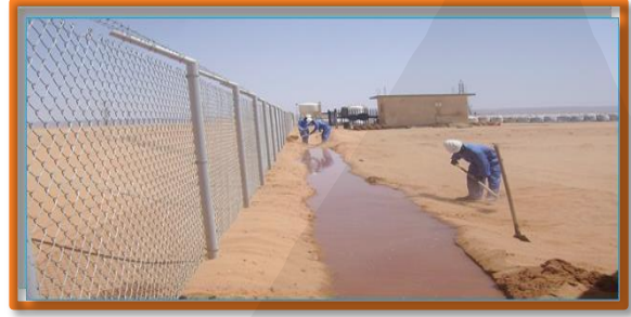
Hand digging and excavation works for UT survey
