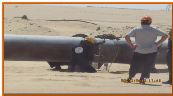
ZOC-103A INSTALLATION SLIP BLIND AT FLARE
